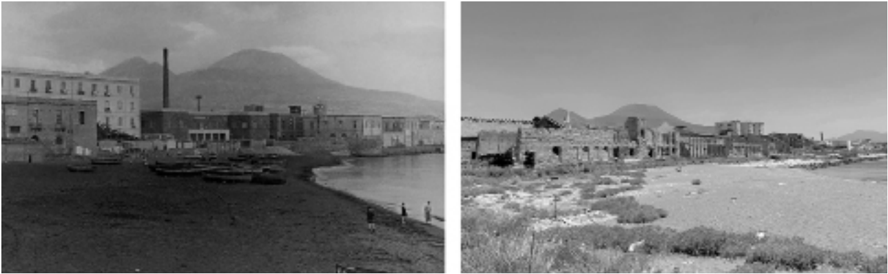
Fig. 5. At the top, views of the Corradini plant during the years of activity, at the bottom, the current state of degradation of the Corradini structures (photographs: D.M. Massari and F. Miranda's thesis).
