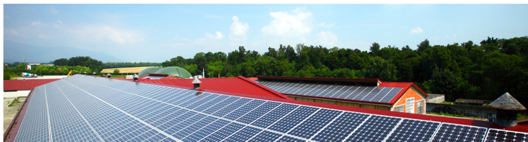
Fig. 1. Existing PV roofs of "La Bellotta".
