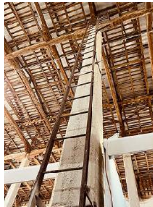
Fig. 8. Reinforced concrete pillar
