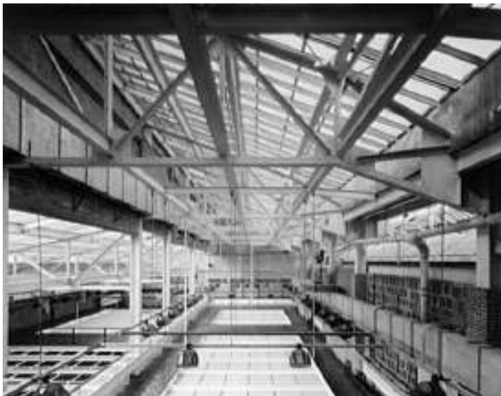
Figure 14. Lighting system between ceiling and roof ( National Gallery of Art. Lighting system between ceiling and roof in National Gallery ), 1950s. National Gallery of Washington D.C. [Source: Library of Congress, Prints & Photographs Division, Theodor Horydczak Collection, (reproduction number, LC-H814-028); ©Library of Congress]
