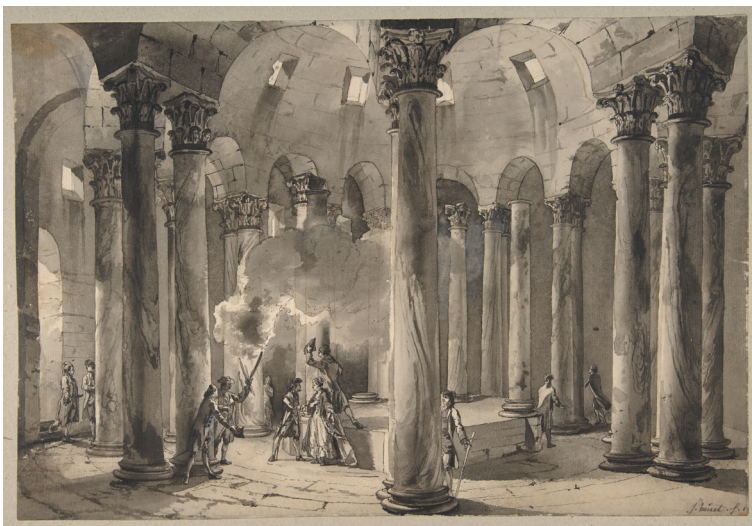
Figure 2 Jean Pierre Louis Laurent Houël, Visitors with Torches Inside a Circular Building (The interior of Santa Maria Maggiore at Nocera Superiore, near Naples) . Ca. 1769. Pen and brown ink, gray-brown wash, heightened with touches of white, over traces of black chalk, 268 × 393 cm. New York, The Metropolitan Museum of Art. © The Metropolitan Museum of Art
