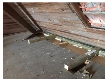
Figure 9. Splice of wooden beams (credits: Aníbal Costa)
