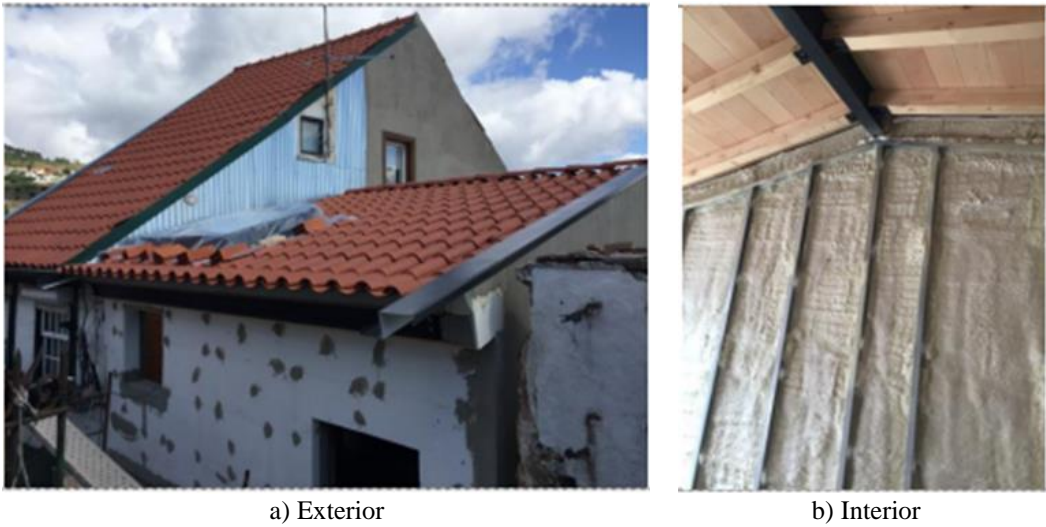
Figure 7. Thermal insulation of walls
