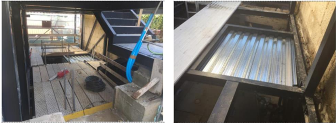
a) Steel stairs
