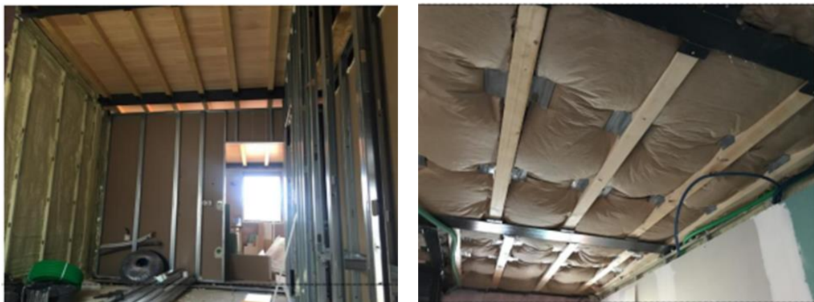
a) Interior partition walls
