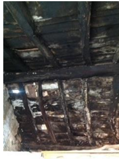
d) Roof in Timber
