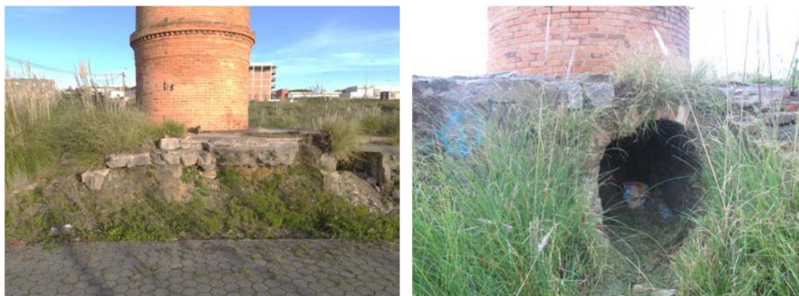
e) Block at the chimney's base
