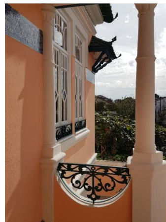
Figure 3. Balcony Cestinhos house (credits: A. Tavares)
