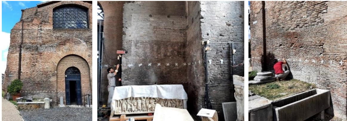
Figure 5. Setup and execution of the sonic testing on the south-east corner pillar of Hall I.
