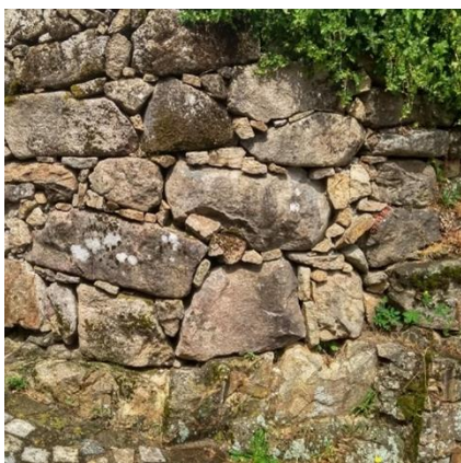
Figure 8. Filling of space in between the big rock with small stone fragments, Porreiras, photo: M. Orszt
