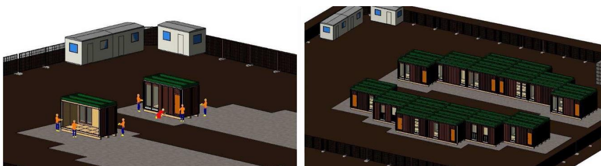
Figure 11. Building phase: modules are placed on the foundation (on the left) and ground floor completed (on the right).
