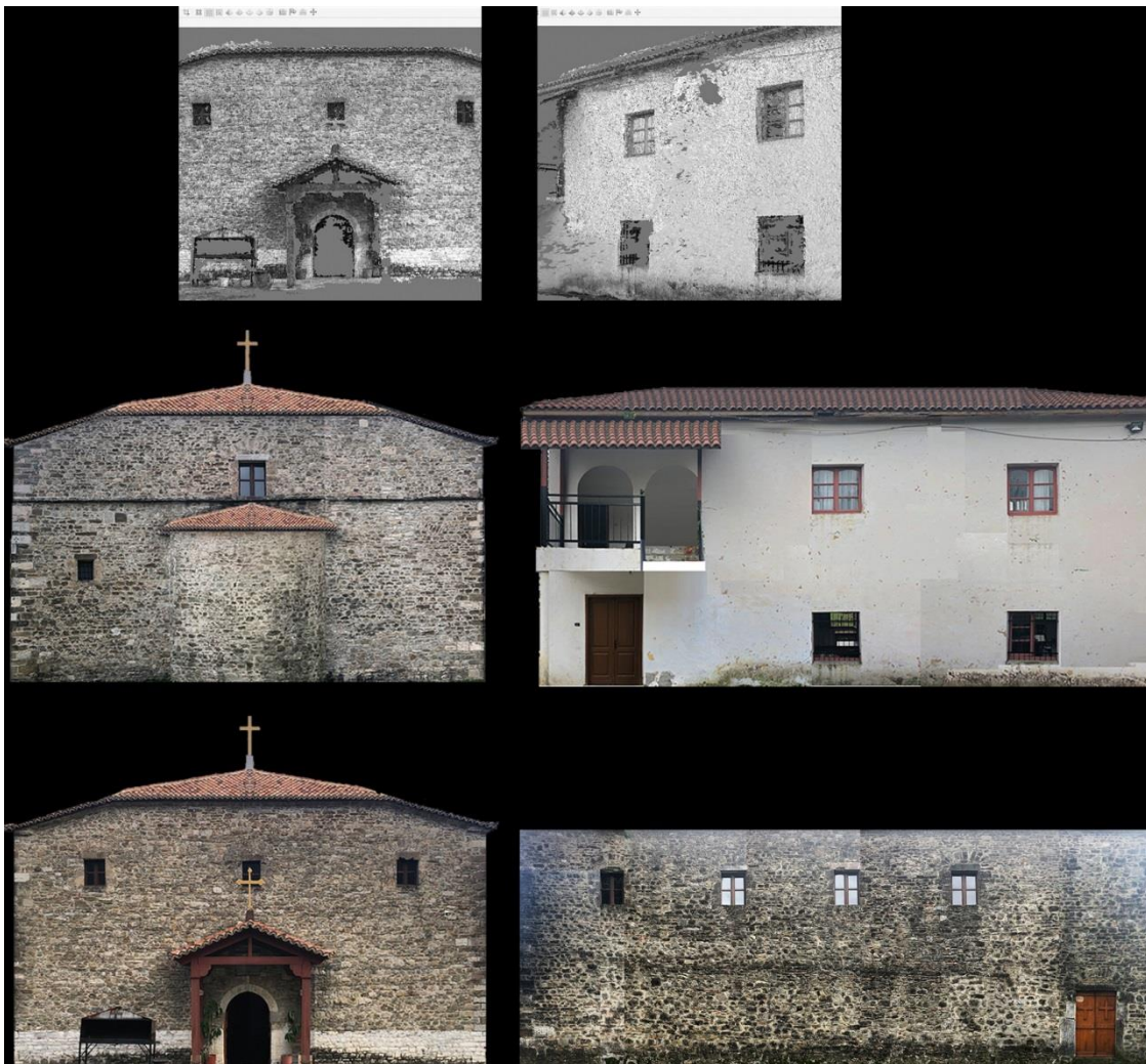
Figure 2. Point cloud processing and orthomosaic generation from photogrammetric survey
