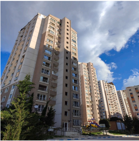
Fig. 1. Intact Concrete Tunnel-Form Buildings after Experiencing Strong Earthquakes and Aftershocks (Turkey, 2023).
