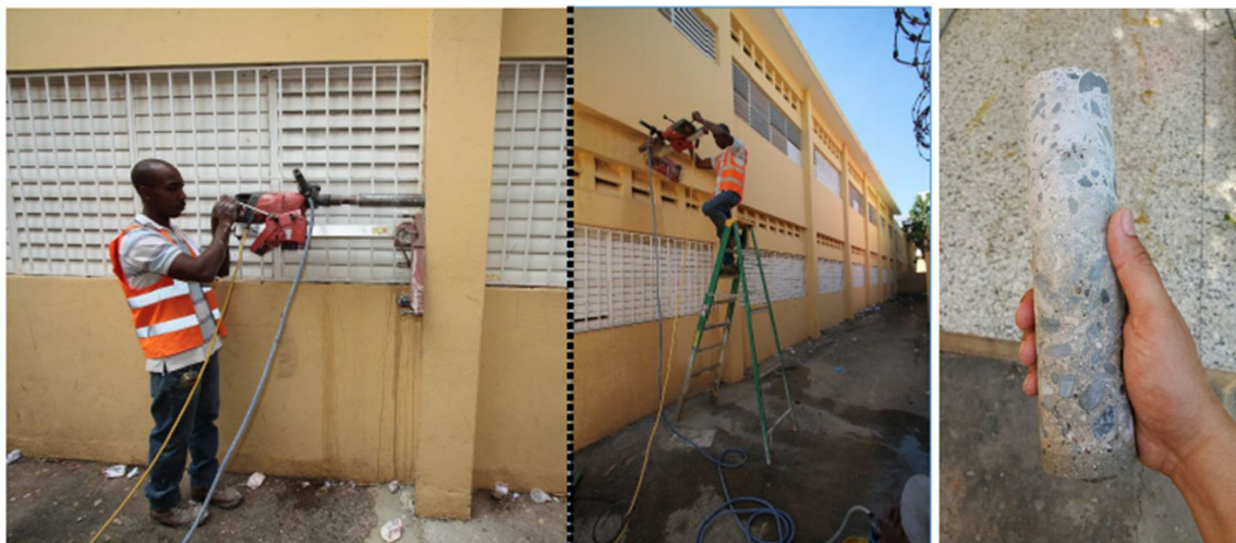
Fig. 15 Concrete core extraction
