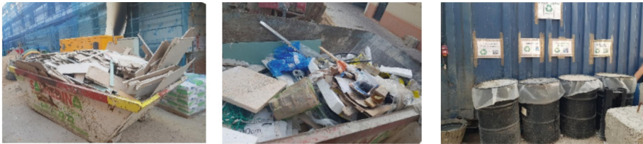
Fig. 1. Vallecas Construction Site (VA001). From left to right: Construction and Demolition Waste (CDW) plasterboard; Non-hazardous mix Level II CDW. Non-stony nature; Hazardous CDW.
