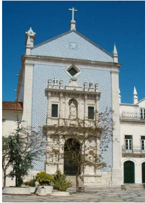
Figure 2. Main elevation of the church.
