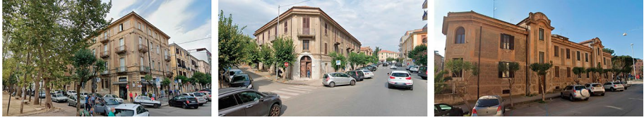
Fig. 7 Some pictures of the studied masonry structures
