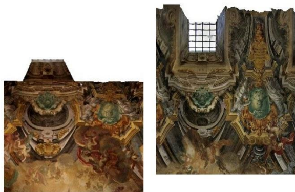
Figure 10. Difference between orthogonal projection and cylindrical projection
