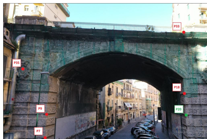
Figure 5. View of the south facade with markers locations. GCPs are represented in red while CP is represented in green.
